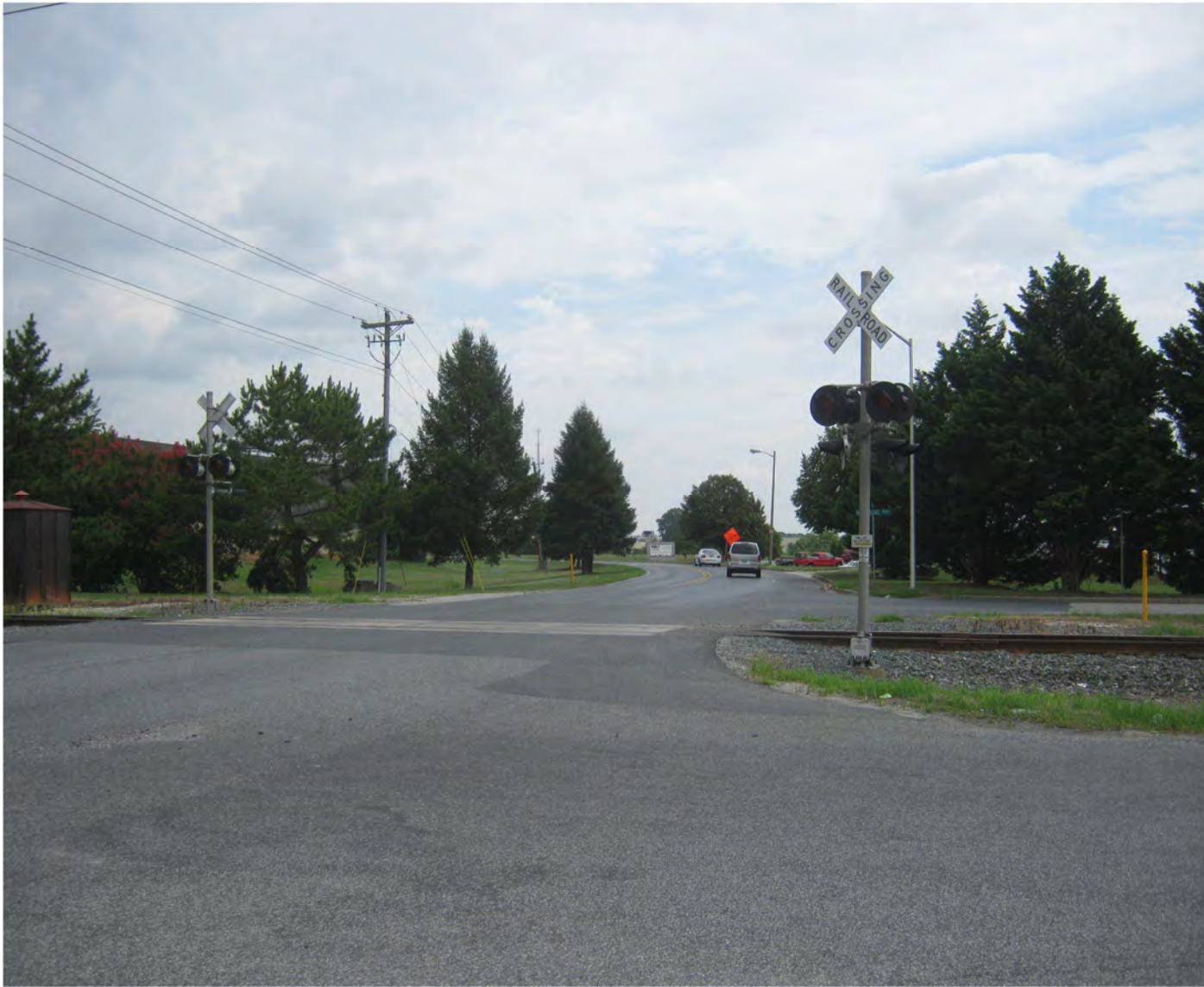
The Naylor Mill Road and Goddard Parkway/Armstrong Parkway intersection has experienced a number of crashes. It is recommended to construct a left run lane on westbound Naylor Mill Road onto Armstrong Parkway and Goddard Parkway to reduce this problem.
