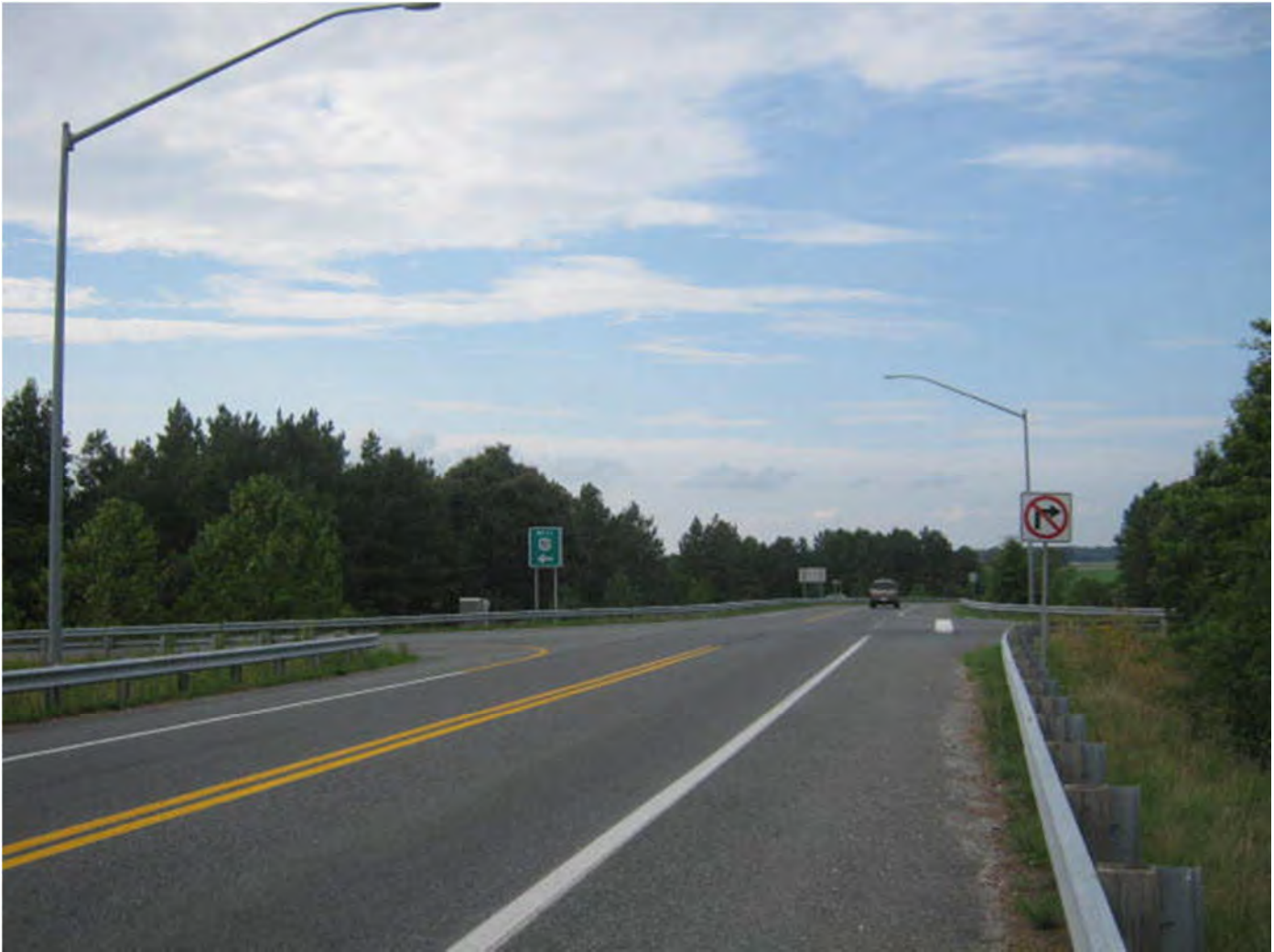
Naylor Mill Road and U.S. Route 50 Westbound Ramp Intersection. Today, this intersection operates well but is expected to experience a poor level of service under future traffic conditions.
